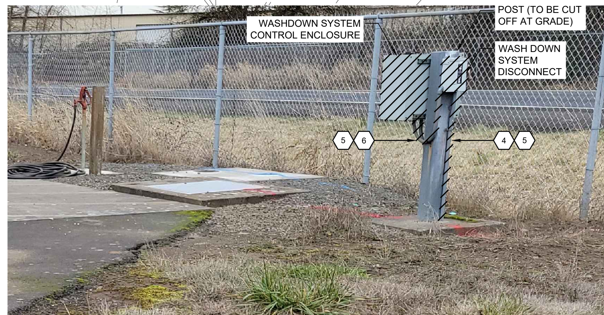
1 - NTS WASHDOWN SYSTEM PEDESTAL DEMOLITION PHOTO DETAIL
