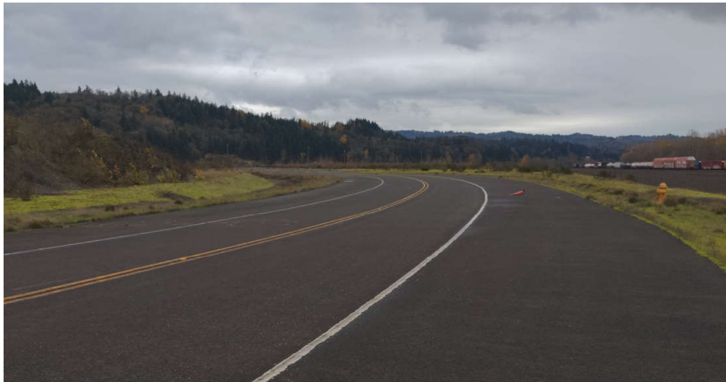
Photo 3: Northern end of Talley Way facing south at the northern end of the study area.
