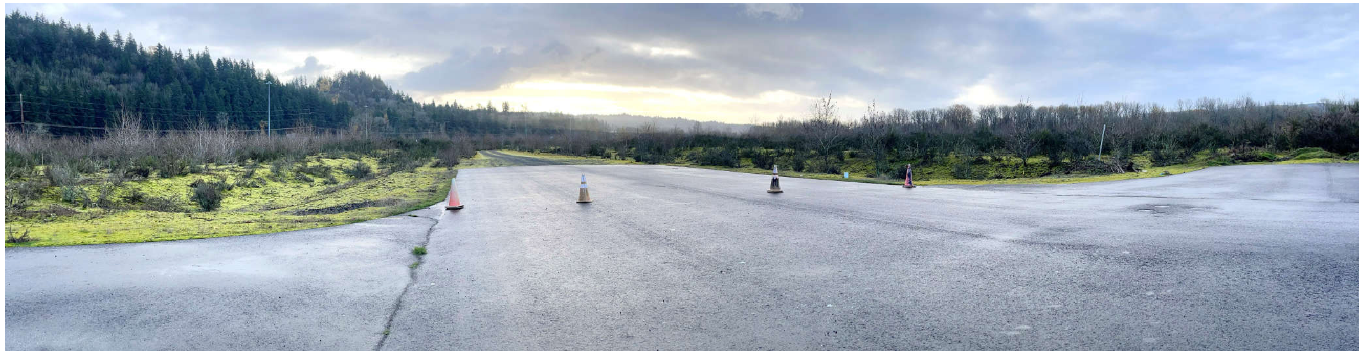
Photo 2: Southern end of Talley Way facing south in the central portion of the study area.
